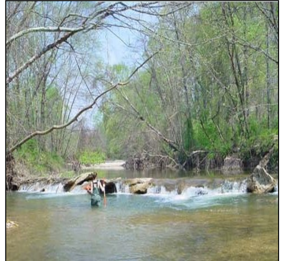
The major fish blockage on Paint Branch, upstream of Route 1 in College Park, Prince George's County, Maryland.
